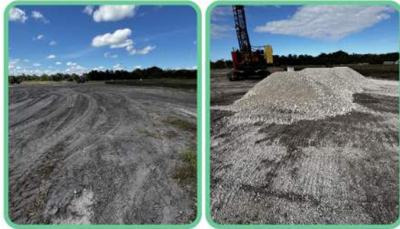
Site Clearing & Onsite Preliminary Construction
