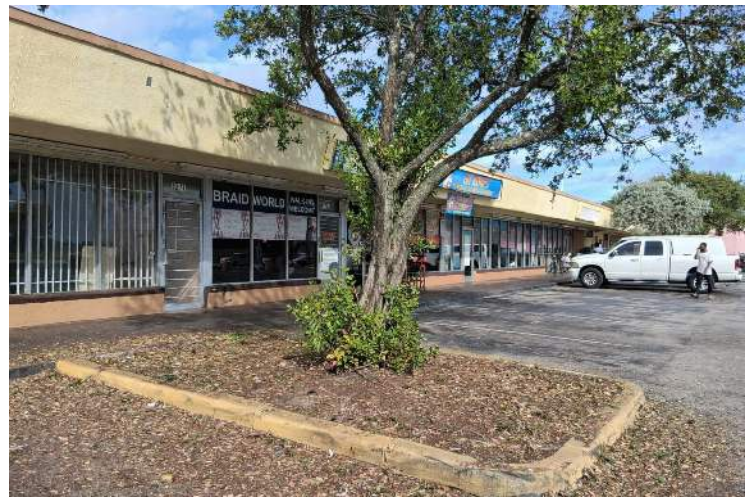
Wyngate Plaza – before completion
