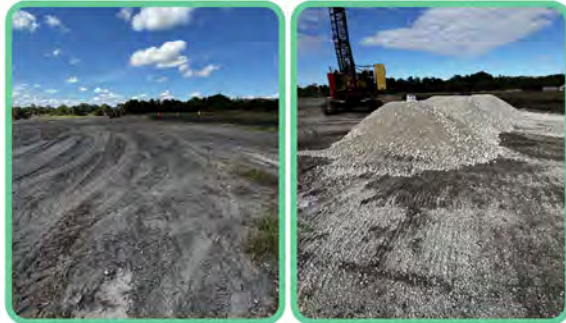
Site Clearing & Onsite Preliminary Construction
